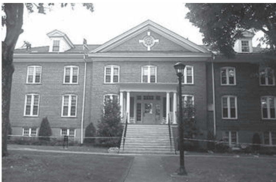
John Wesley Hall, the administration building, having its roof repaired.
