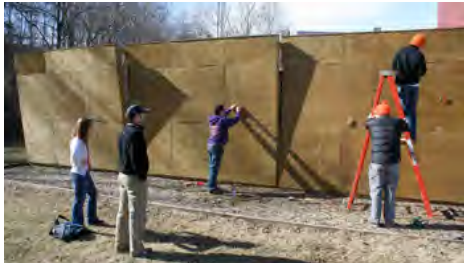
Bouldering wall construction progressing.
